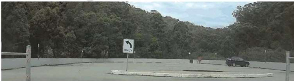
Figure 3-18: Underutilised upper deck car park
