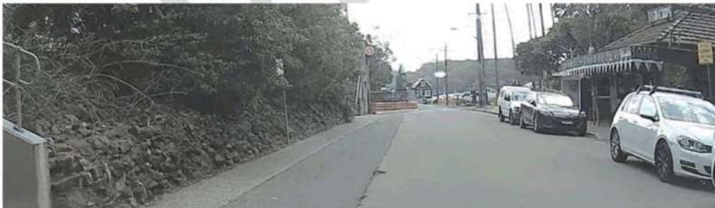
Figure 3-8: No Parking sign obstructed by foliage outside Hawkesbury River Station
