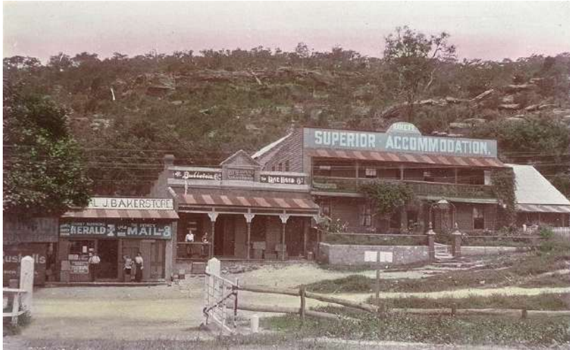
This postcard by William Broadhurst dates from about the end of World War I. It shows Baker's three business premises. The middle one had a top storey added to it and it is one of Brooklyn's oldest buildings.
