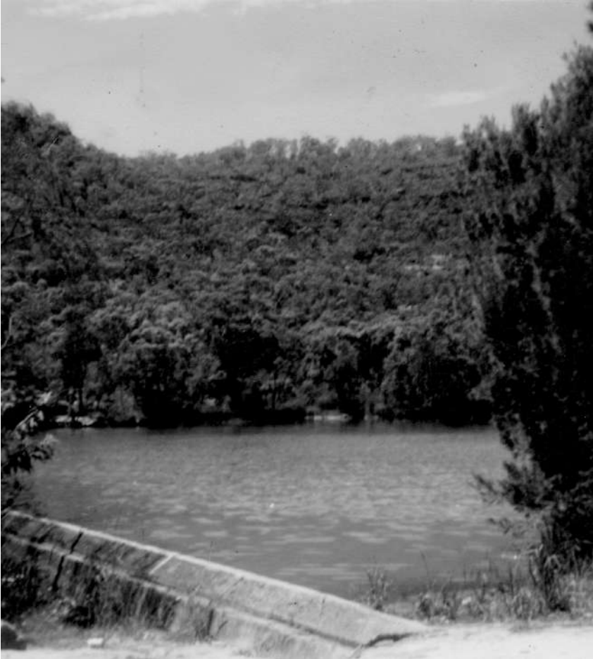
The old railway reservoir, high in the hills behind Brooklyn. The height of the wall has been reduced by National Parks for some reason that it best knows. It still remains an attractive stretch of water in beautiful surrounds.
